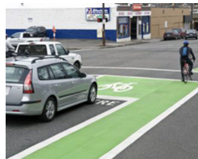
Painted and striped bicycle box at a signalized intersection
